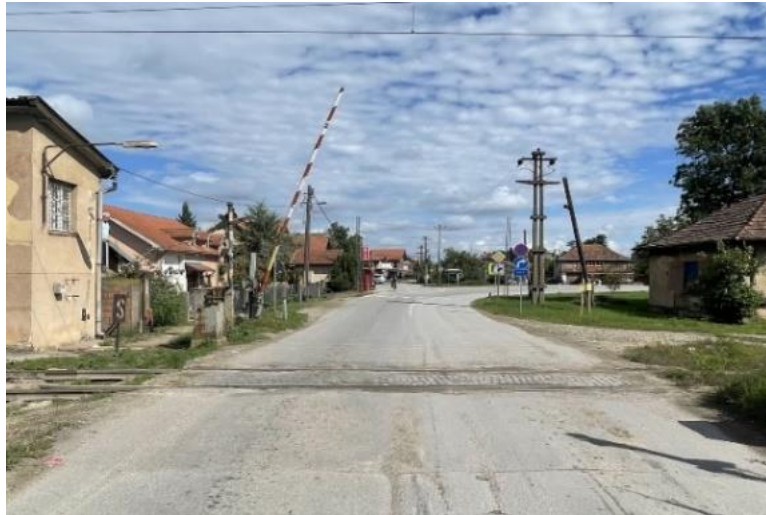
Figure 12: Existing RLC before reconstruction
