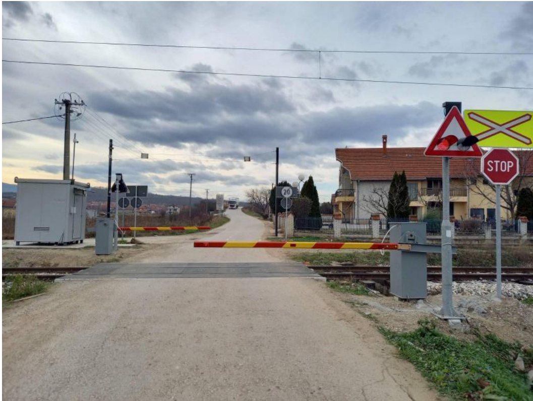
Figure 1: Existing RLC light signal
