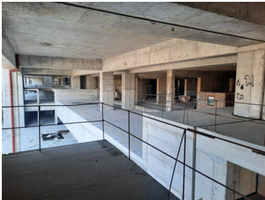
Figure 2. Constructed premises and area under slab where the Project will be located-inside view
