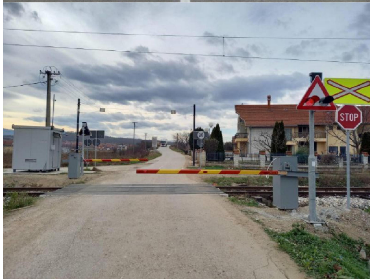
Figure 12: Example of a RLC after reconstruction
